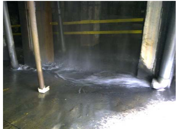
Figure 4: Water Flow under the Presses
