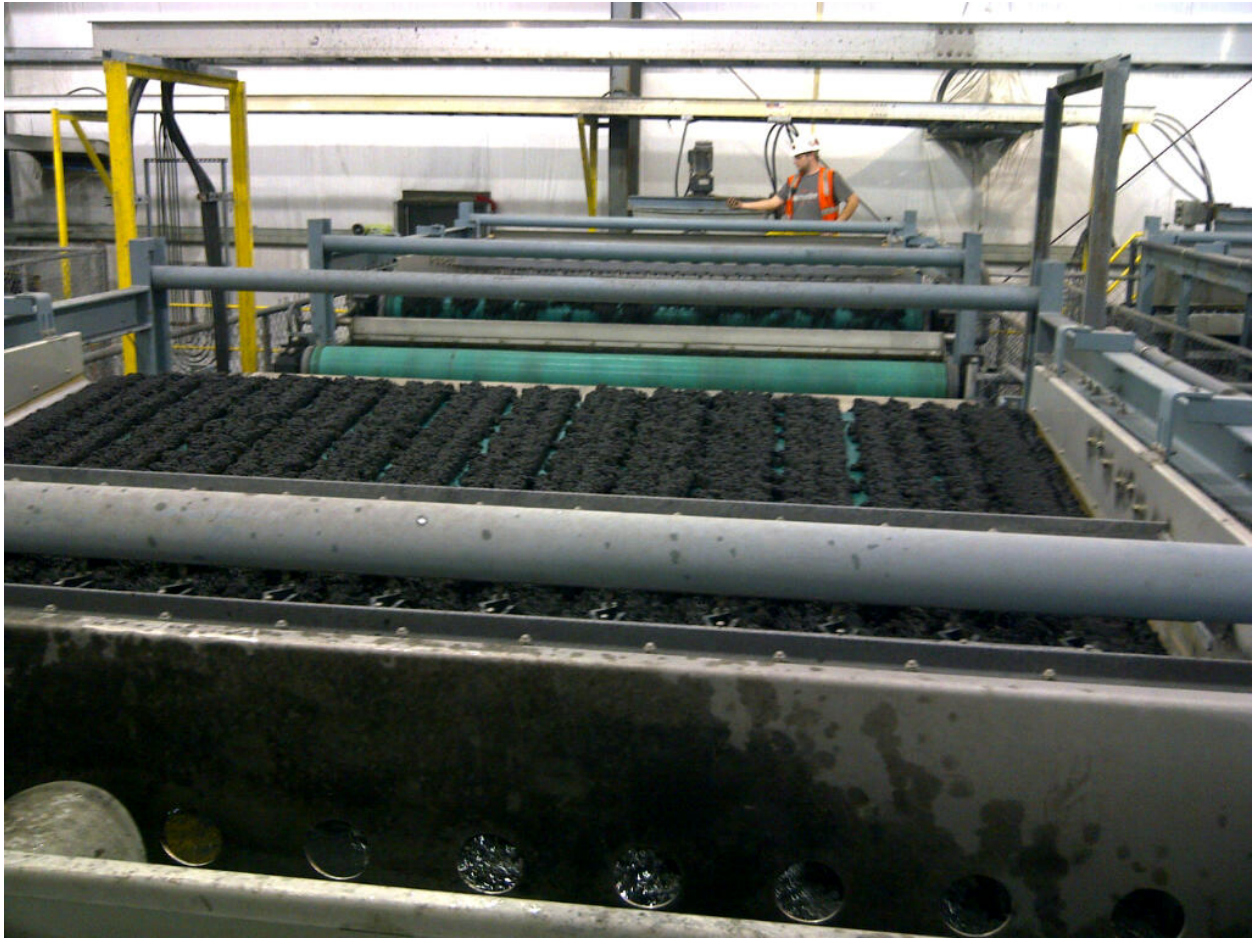
Figure 9: Tailings Solids on the Top Belt of the Press
